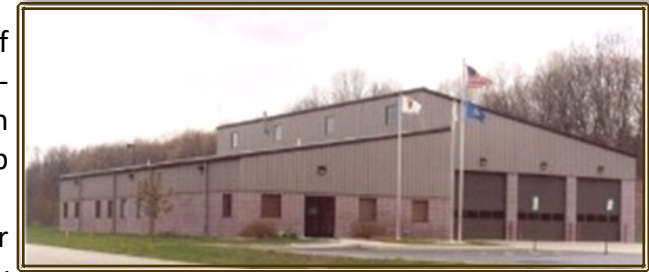
Fire Station 2 - 3500 South 6th Street: Built in 2000
