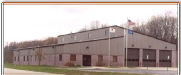
Fire Station 2 - 3500 South 6th Street: Built in 2000
