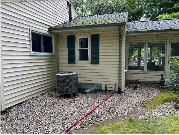
Looking north at the residence and breezeway.
