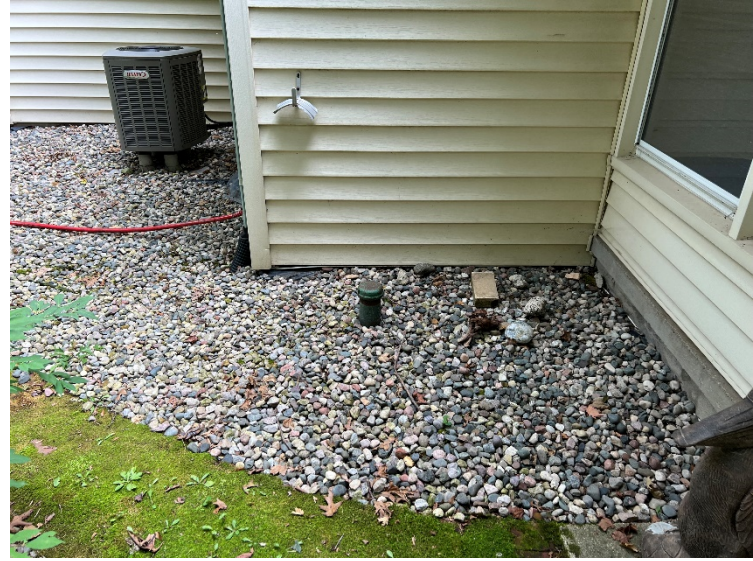
Closeup view of potential fill port.
