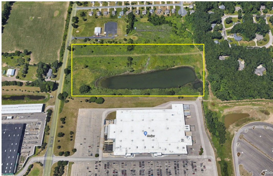
Figure 2: Site Aerial: 9 th Street (Parcel 05-14-130-017)
