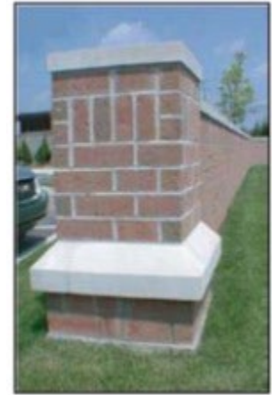
A street wall used to screen the adjacent parking lot.
