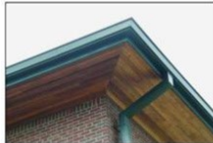
A large overhanging eave with a wood soffit is above.
