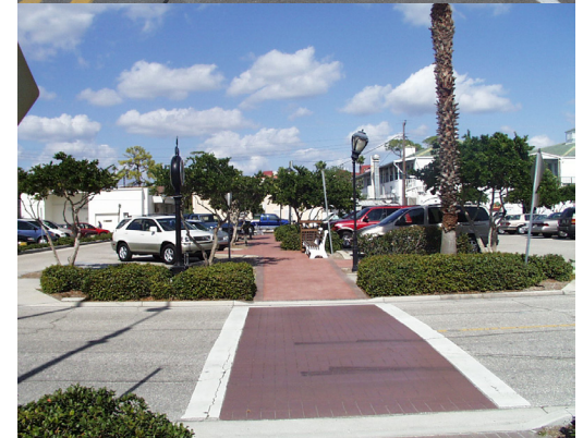
Pedestrian refuge island (top) and designated crosswalks with contrasting materials (bottom) are recommended pedestrian safety improvements
