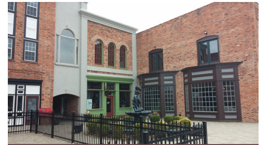
Unique site features, such as public art, are encouraged to be incorporated into new development within the village
