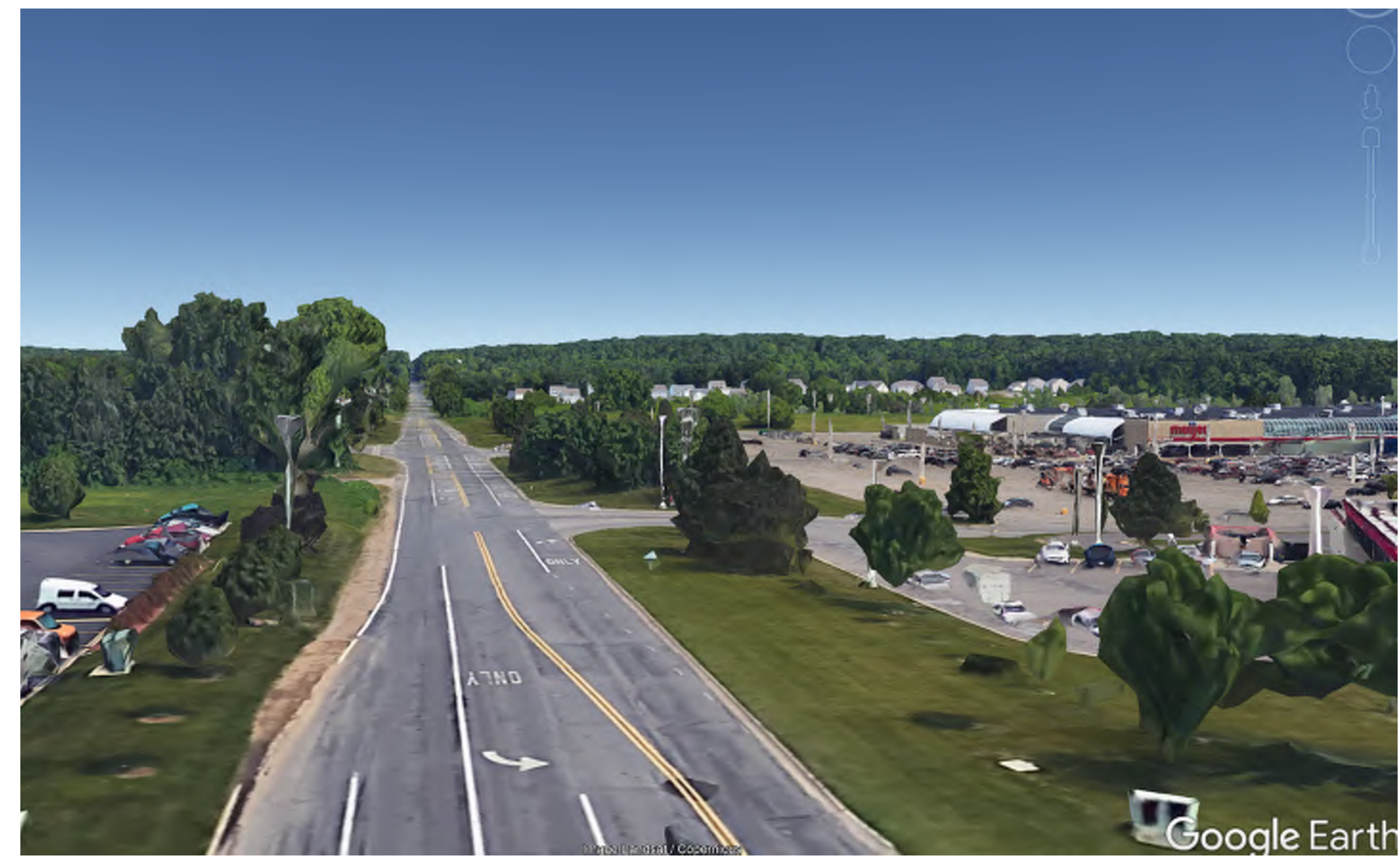
LOOKING DOWN 9TH STREET
