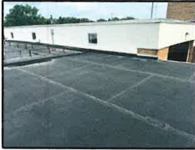
EXISTING ROOFING SYSTEM:
