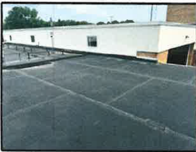
EXISTING ROOFING SYSTEM:
