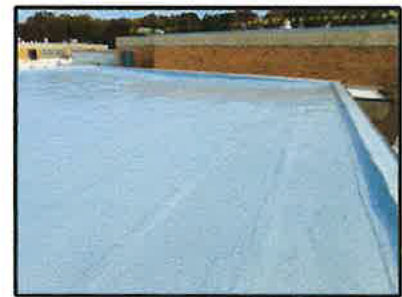
NEW ROOFING SYSTEM:
