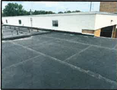
EXISTING ROOFING SYSTEM:
