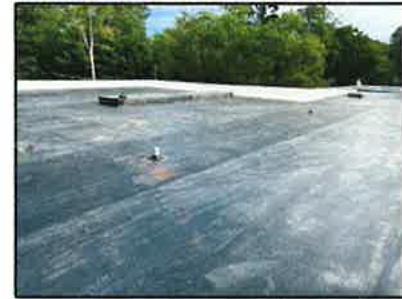
NEW ROOFING SYSTEM:
