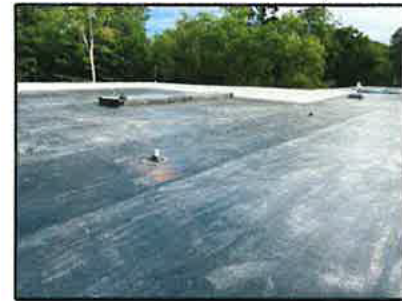
NEW ROOFING SYSTEM:
