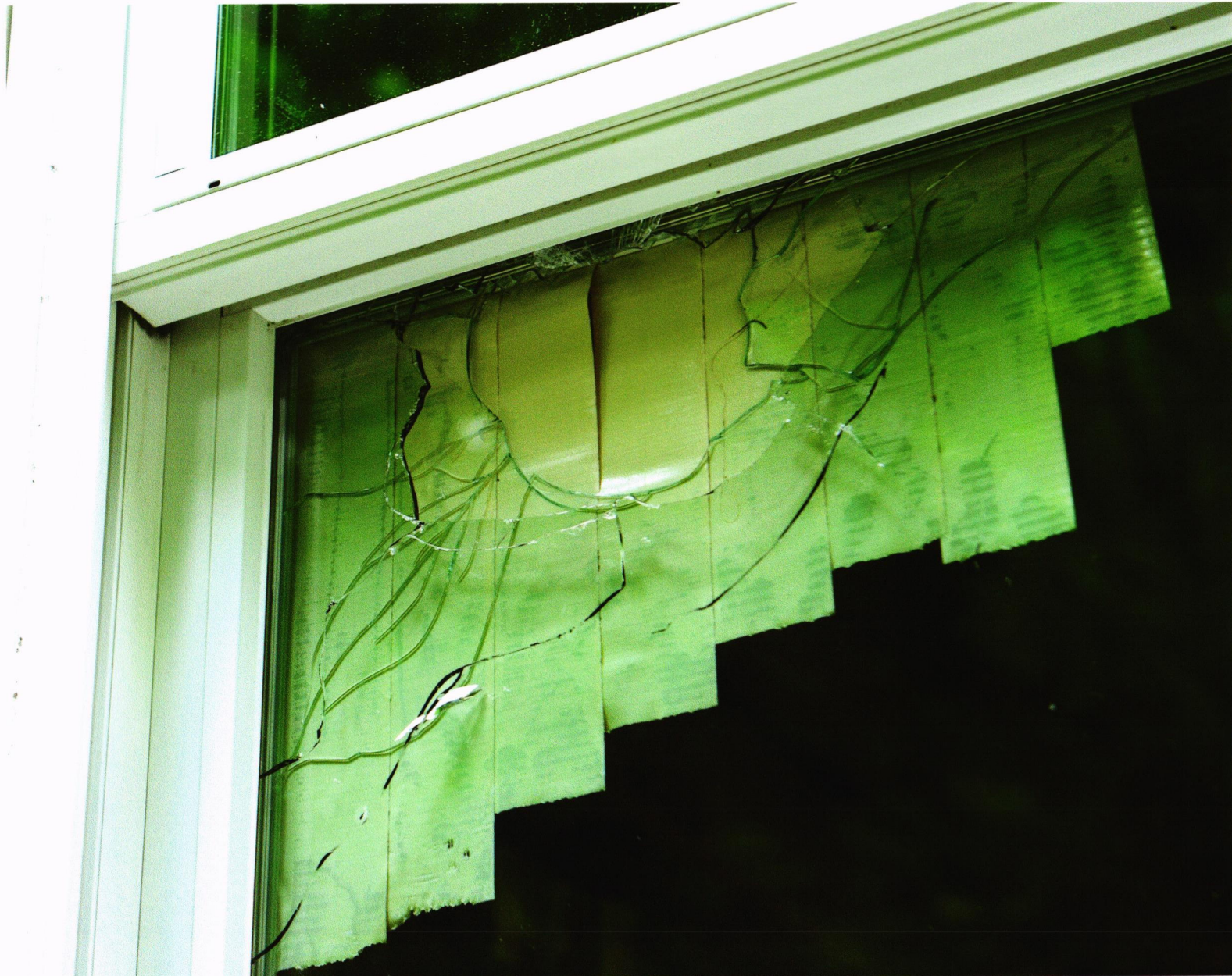
One of the Four East Facing Windows
