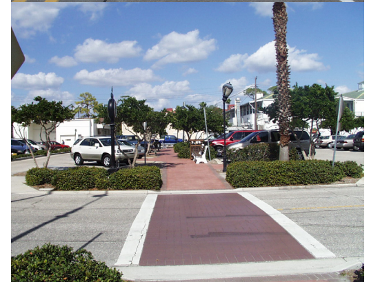
Pedestrian refuge island (top) and designated crosswalks with contrasting materials (bottom) are recommended pedestrian safety improvements
