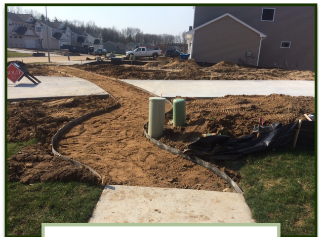
Sidewalk Installation Inspection
