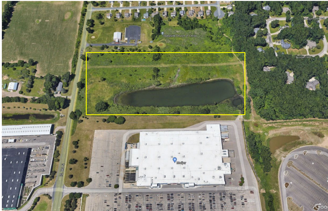
Figure 2: Site Aerial: 9 th Street (Parcel 05-14-130-017)
